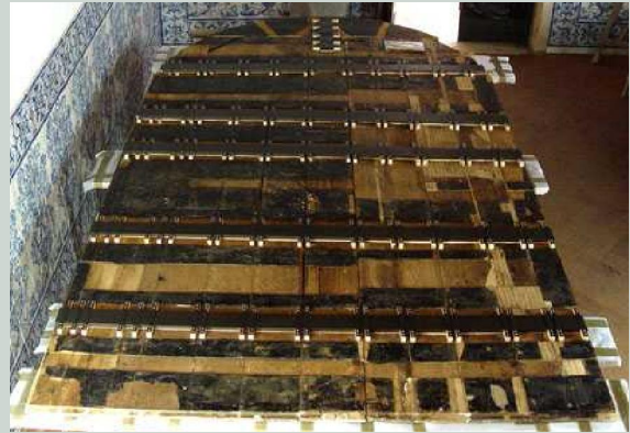
Figure 18. Detail of the new reinforcement system with cross aluminum bars.
