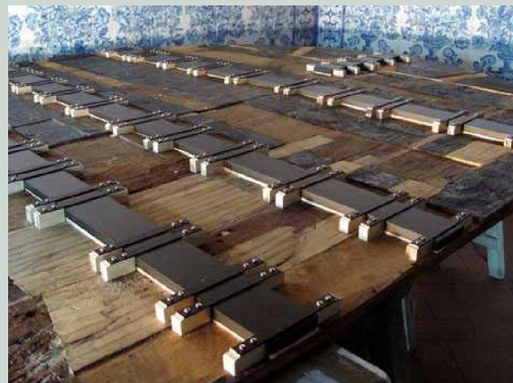
Figure 17. The new reinforcement system with cross aluminum bars.
